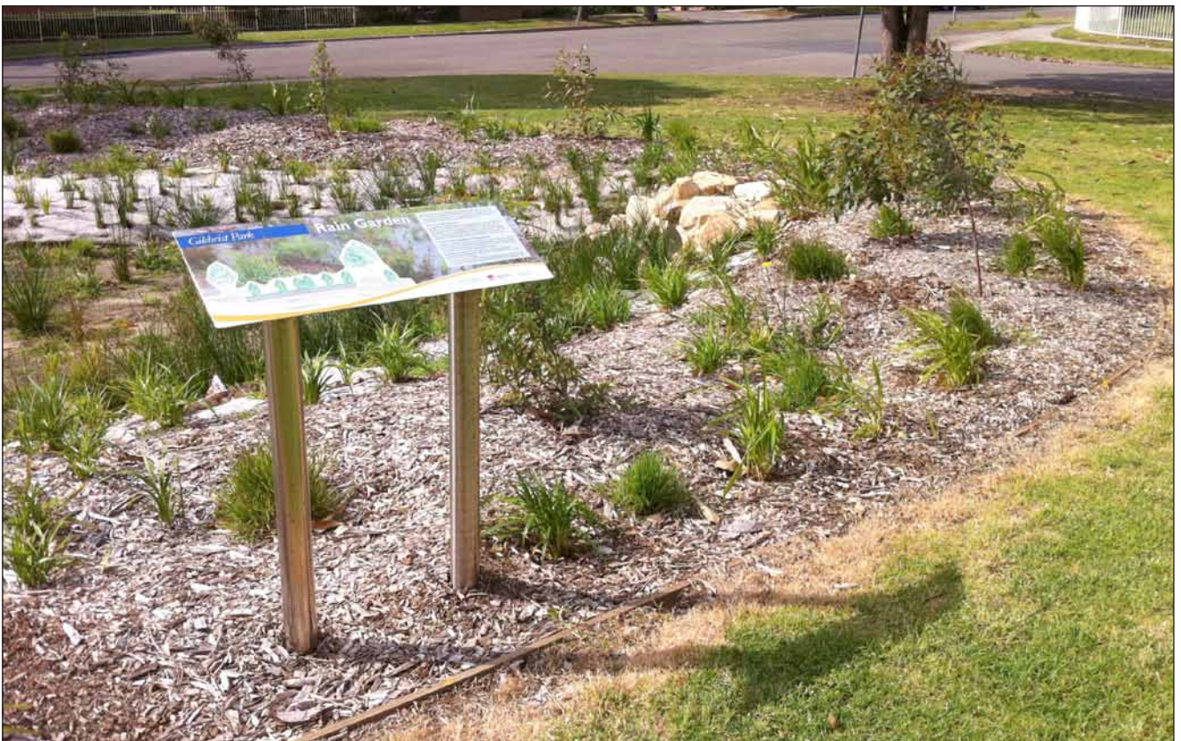
Figure 3.4 – Photo of Gilchrist Park Rain Garden in Bexley North. An example of water sensitive urban design in practice to improve the quality of stormwater.
